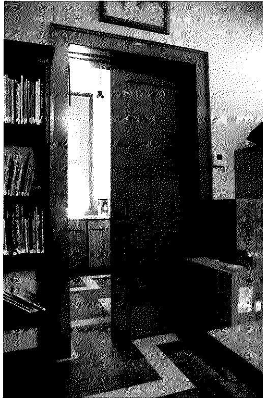
Image 10: Interior, Hartington Carnegie Library, pocket door from historic reading room to workroom; camera facing south.
