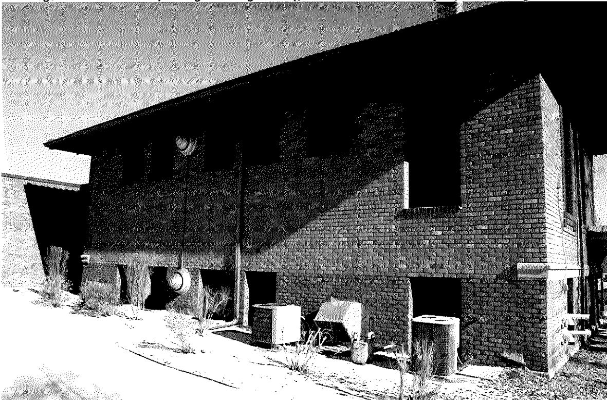
Image 03: West façade, Hartington Carnegie Library with southwest side of addition; camera facing northeast.
