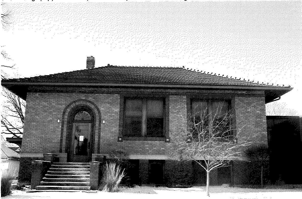
Image 01: East façade, Hartington Carnegie Library with hyphen to addition; camera facing west.
