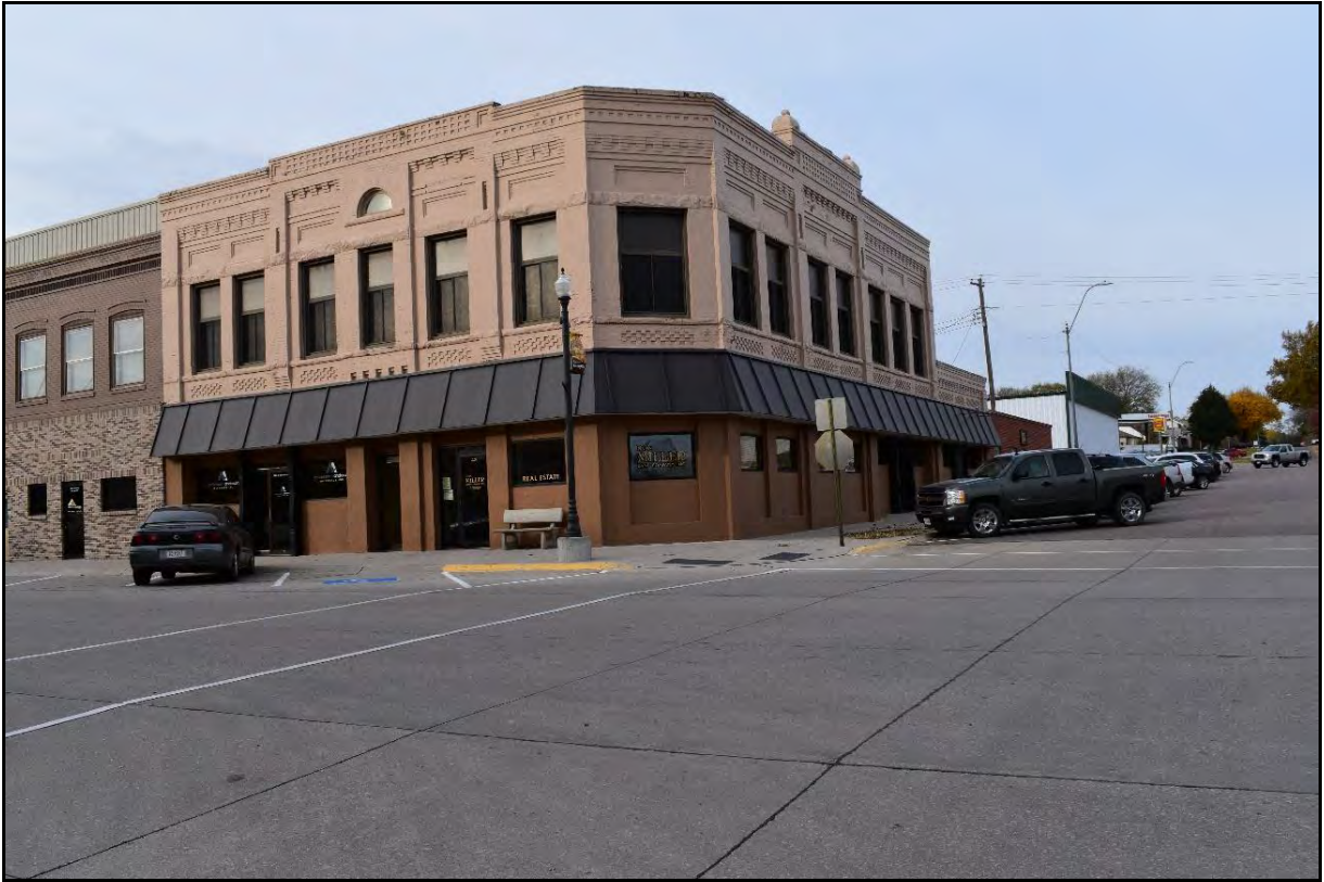
Photograph 15: 226 North Broadway (North and East Façades), Camera Facing West
