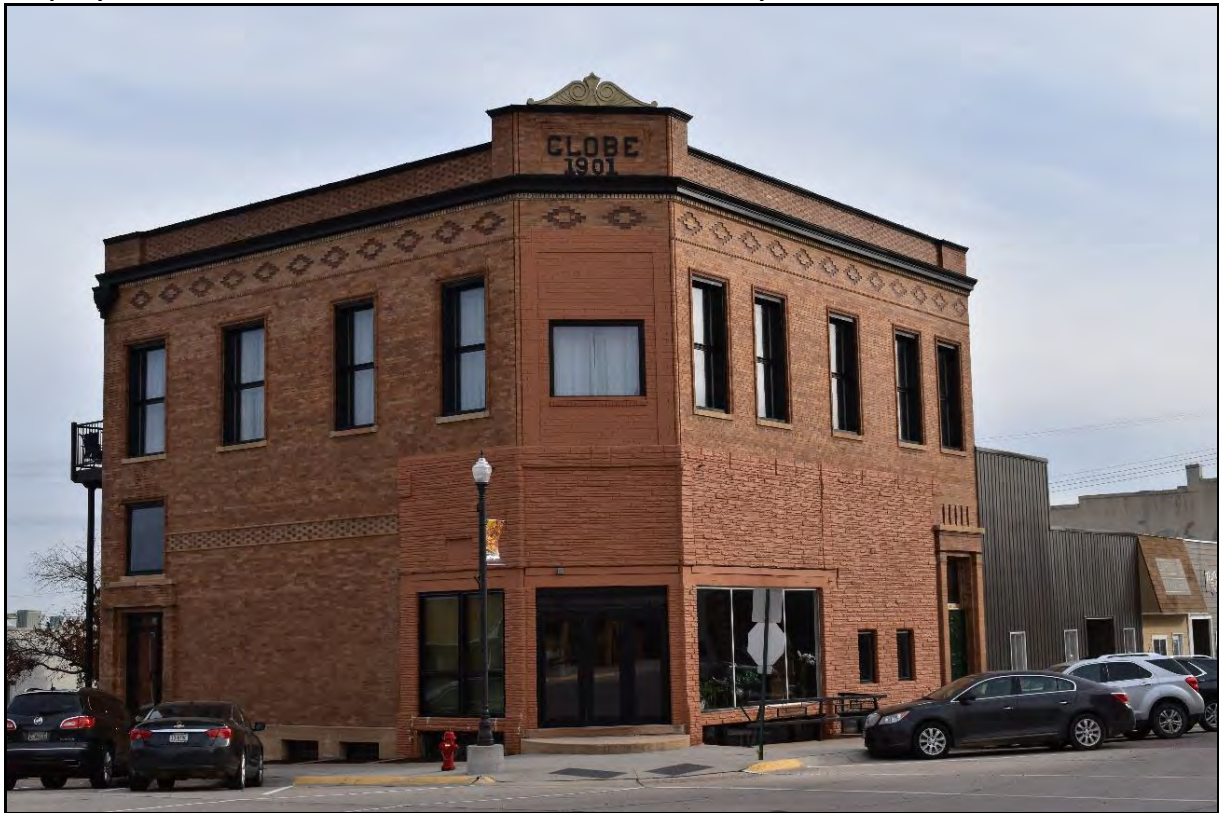
Photograph 17: 301 North Broadway (South and West Façades), Camera Facing Northeast
