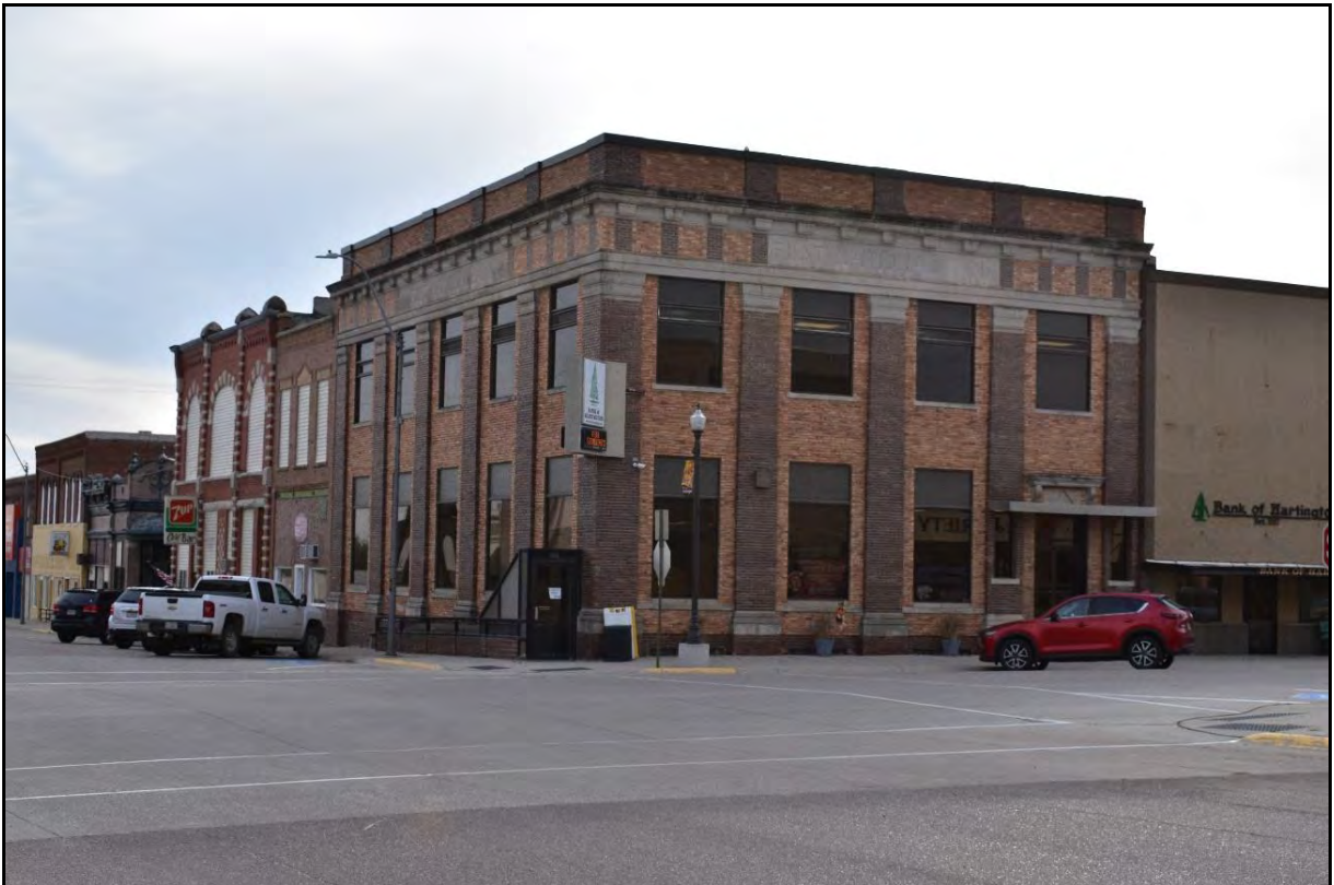
Photograph 16: 229 North Broadway (North and West Façades), Camera Facing Southeast
