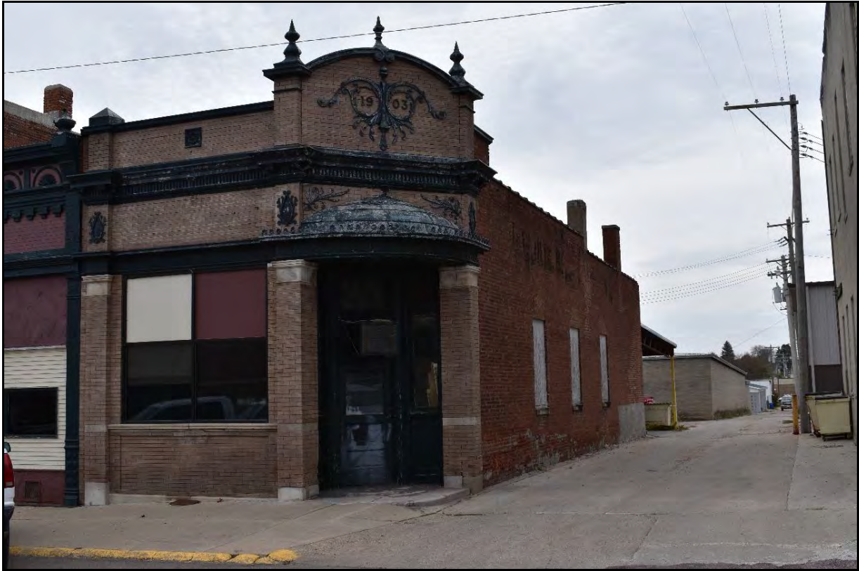
Photograph 23: 109 A East Main (North and West Façades), Camera Facing South
