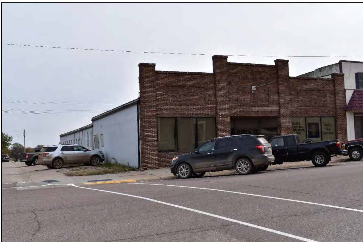
Photograph 18: 321 North Broadway (North and West Façades), Camera Facing East
