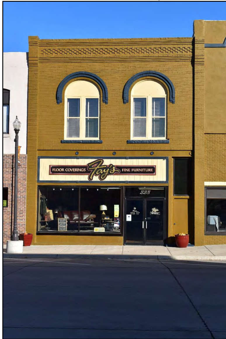
Photograph 14: 223 B North Broadway (West Façade), Camera Facing East
