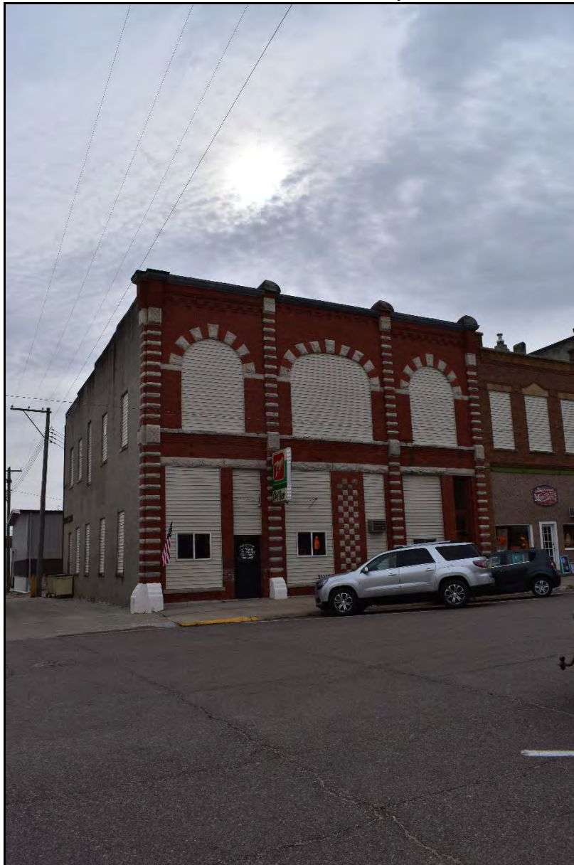
Photograph 22: 107 East Main (North and East Façades), Camera Facing Southwest
