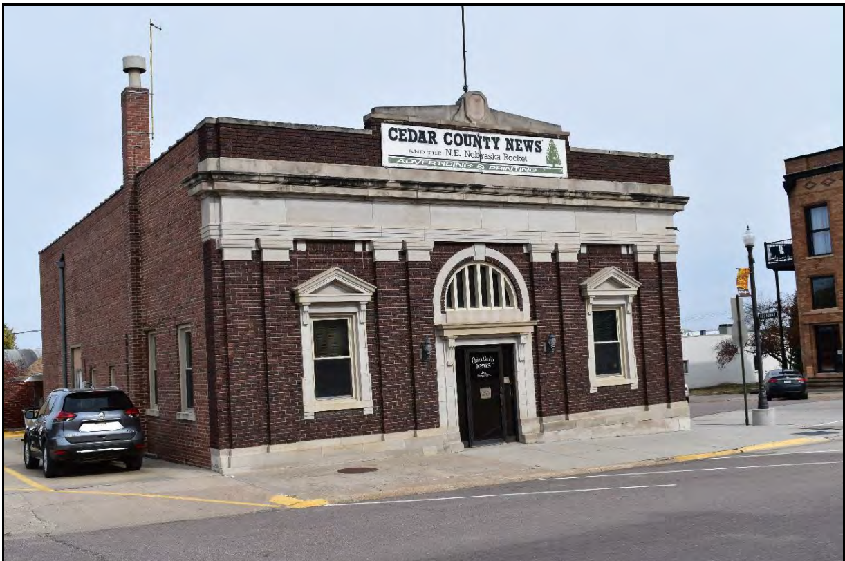
Photograph 20: 102 West Main (South and West Façades), Camera Facing Northeast
