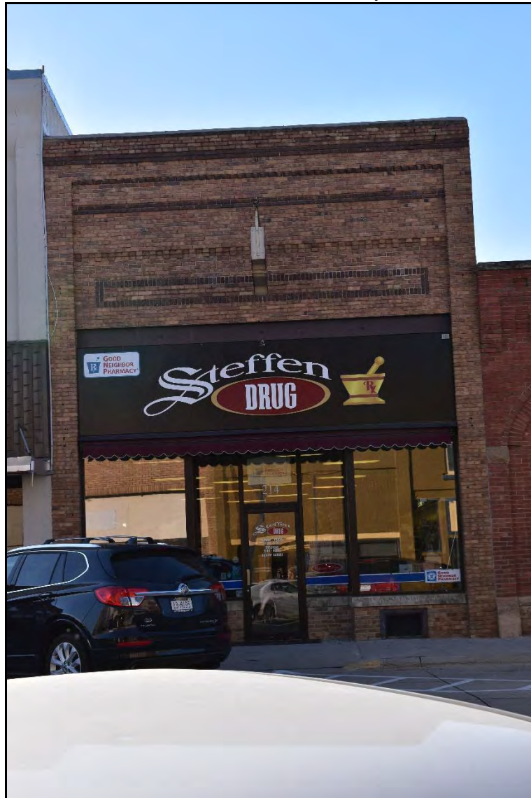
Photograph 13: 214 North Broadway (East Façade), Camera Facing West
