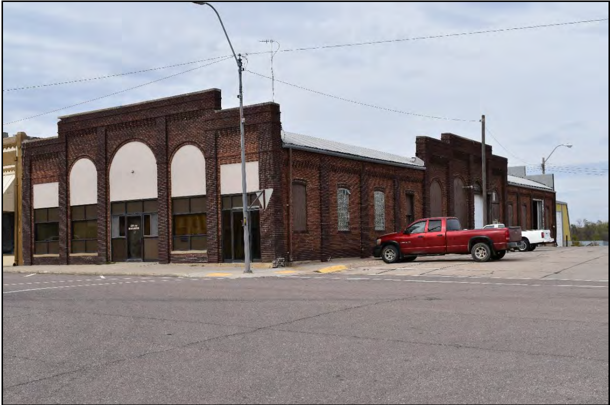
Photograph 21: 124 East Main (South and East Façades), Camera Facing Northwest
