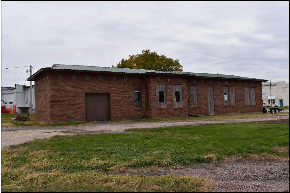
Photograph 19: Train Depot (Northeast and Southeast Façades), Camera Facing Southwest
