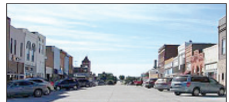
Downtown Street Improvement Project Completed 2013
