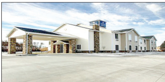
Cobblestone Inn & Suites (2013) Project by local investors Includes 29 rooms, meeting room, weight room, lounge area,
