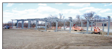
New Firehall Currently Under Construction
